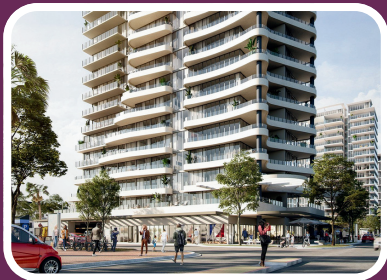
Construction of multistoried buildings
