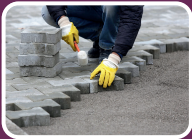
Gravel and Concrete Paving
