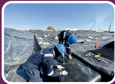
HDPE Lining Work
